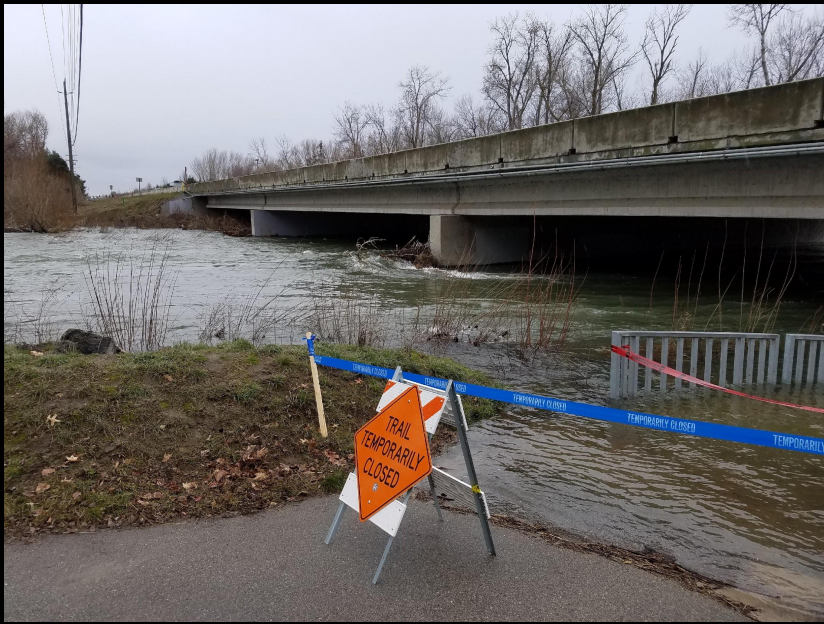
Boise River Flooding (2017)
